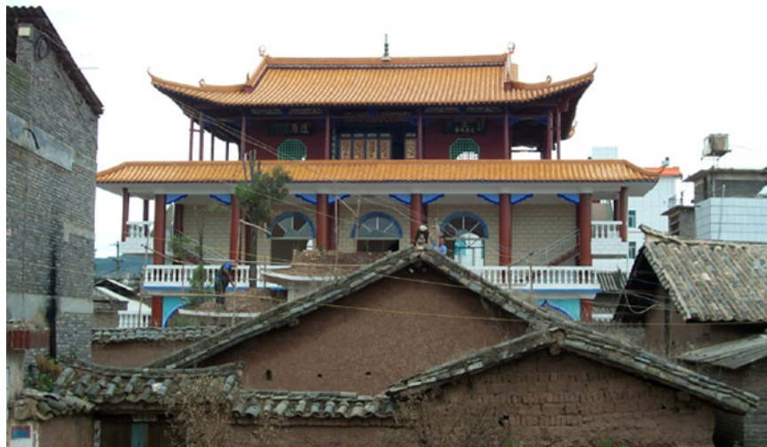
FIGURE 7: YAO'AN CITY NEW MOSQUE, FRONT VIEW.
