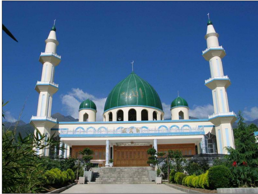
FIGURE 5: DALI CITY NEW MOSQUE.
