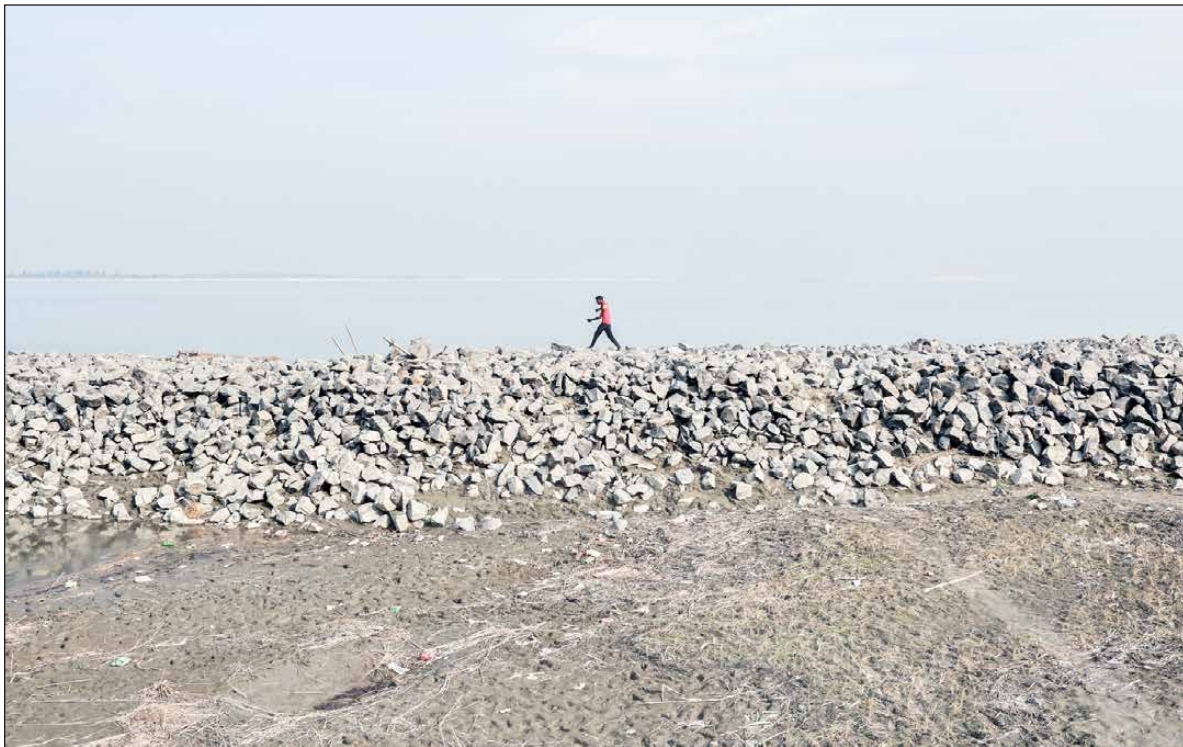
Figure 20. An embankment at the Padma River that protects the town of Sirajgonj. Location: Jamuna River, Sirajgonj, Bangladesh Date: 20 December 2014
